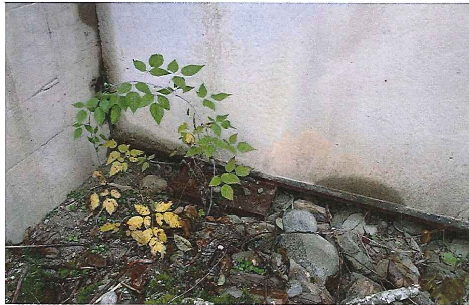
CK2114 Left Abutment Bearing
