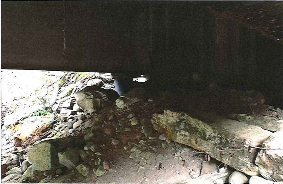
CK2114 Right Abutment
